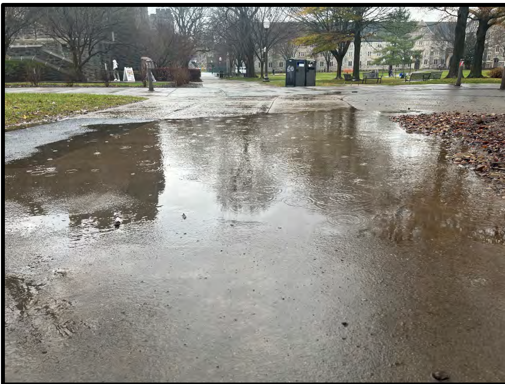
Figure 3. Path blocked by pooled rainwater.
